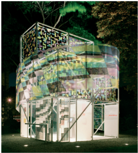
ill. Energy.13.1, ill. Energy.13.2 Smart Wrap (patent pending) by Kieran Timberlake investigates the idea of an off-the-roll material consisting of OLED (light), PCM (climate) and flexible solar modules (energy), continuously manufactured using combined lamination and printing processes, which combines all the important functions of a building envelope.
