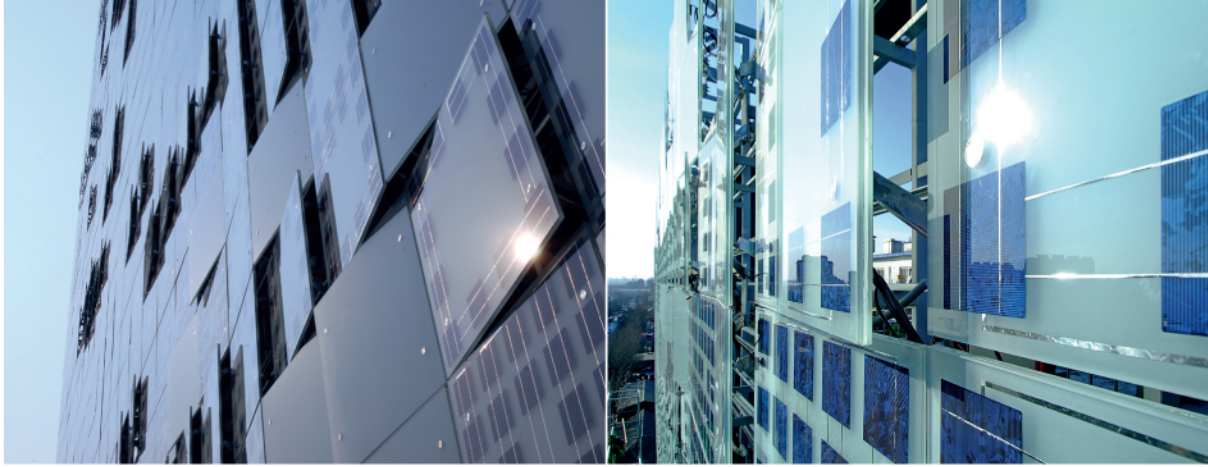
ill. Light.04.1, ill. Light.04.2, ill. Light.04.3 GreenPix—Zero Energy Media Wall by Simone Giostra & Partner with Ove Arup. LED media façade with integrated solar panels. The electricity required to operate the LEDs at night is generated by converting sunlight during the day. • See Light.04, p. 168
