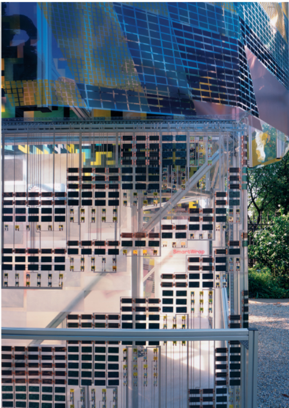
ill. Energy.13.1, ill. Energy.13.2 Smart Wrap (patent pending) by Kieran Timberlake investigates the idea of an off-the-roll material consisting of OLED (light), PCM (climate) and flexible solar modules (energy), continuously manufactured using combined lamination and printing processes, which combines all the important functions of a building envelope.
